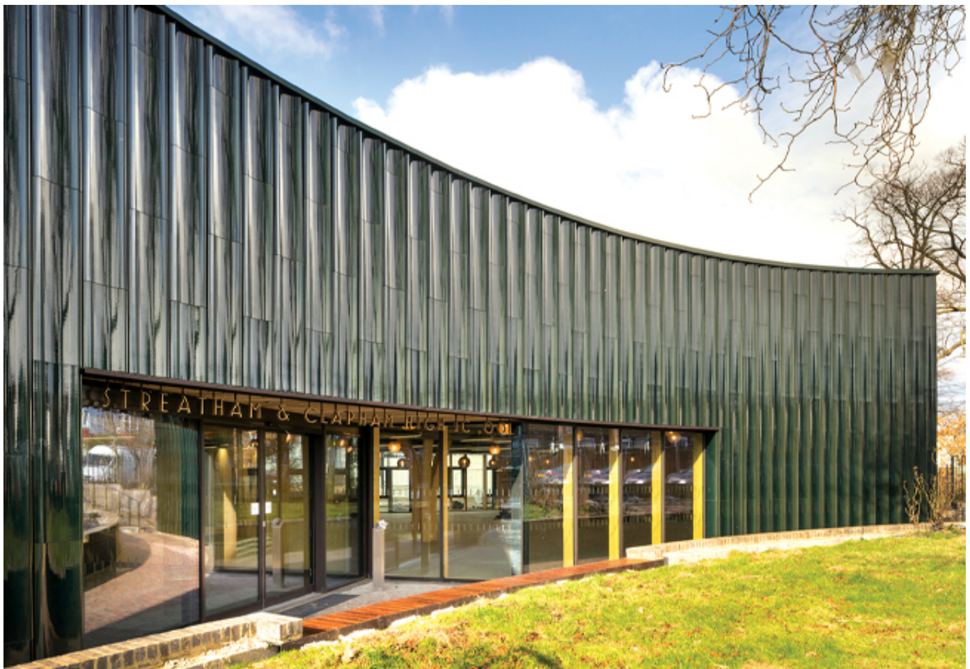
The ground-floor extension includes a new dining hall, kitchen, reception and school entrance
