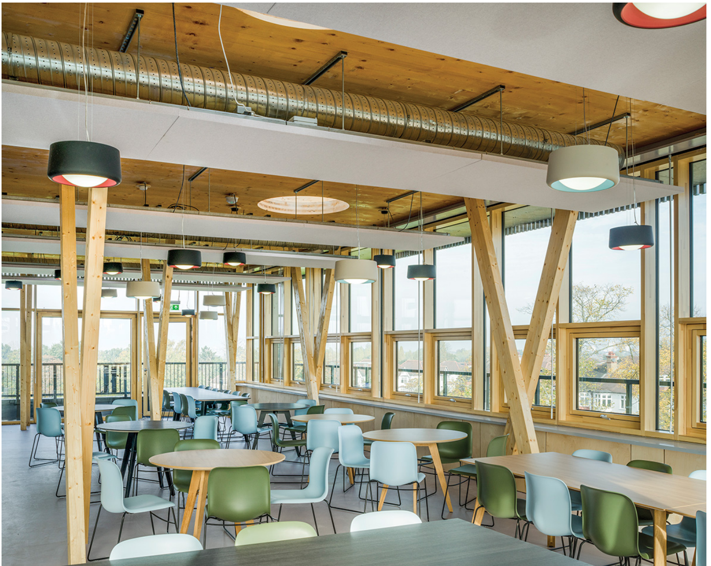
Exposed CLT gives the school's new dining room a warm, natural look
