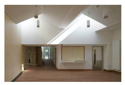
The architects recycled the existing steel structure, concrete slab and masonry walls of the pre-existing building and added a double pitched facade that bows down to open a view to the stained-glass window of the vestry behind.
