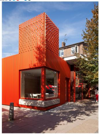
The striking red facade of East Street Exchange was created using ano dised aluminium. Anodisation is a chemical process that makes aluminium more durable, and allows it to be dyed a different colour.
